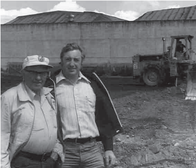
Bill Etchegoin and Jean Gorostaigue at the construction site of “the future home of the Basques”. Photograph courtesy of San Francisco Urazandi Collection.
